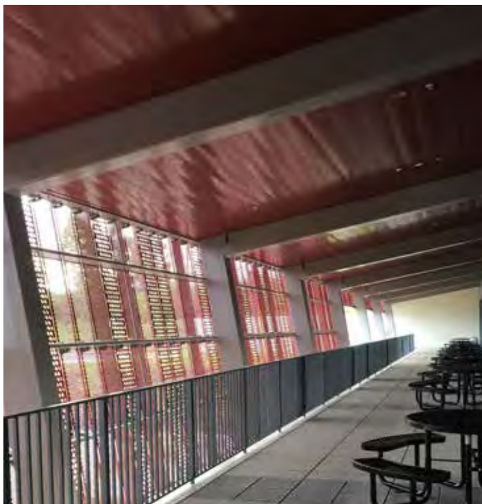
The second-floor lanai, is protected from the elements by a perforated outer wall and exposed steel framing that is a contemporary interpretation of the thatched framing of a traditional Hawaiian hale.
